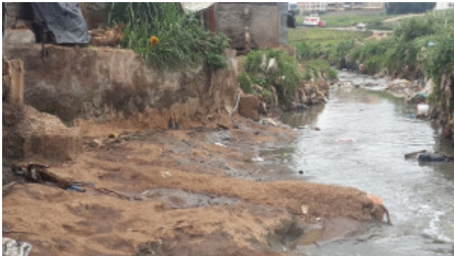
Sewage drains from pit latrines directly into the Motoine River in Kibera, Kenya. Photo: Nicholas Kiulia.
